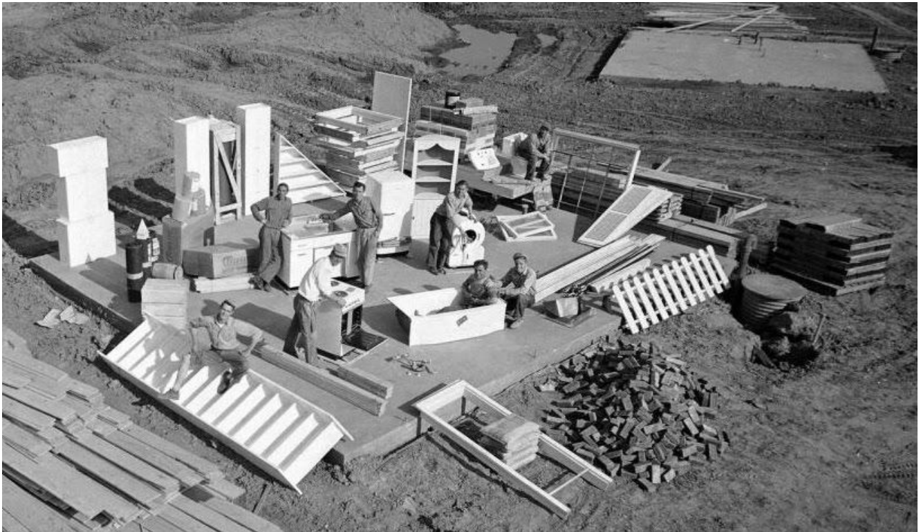
above: construction materials delivered to a Levittown site after foundation poured 7
